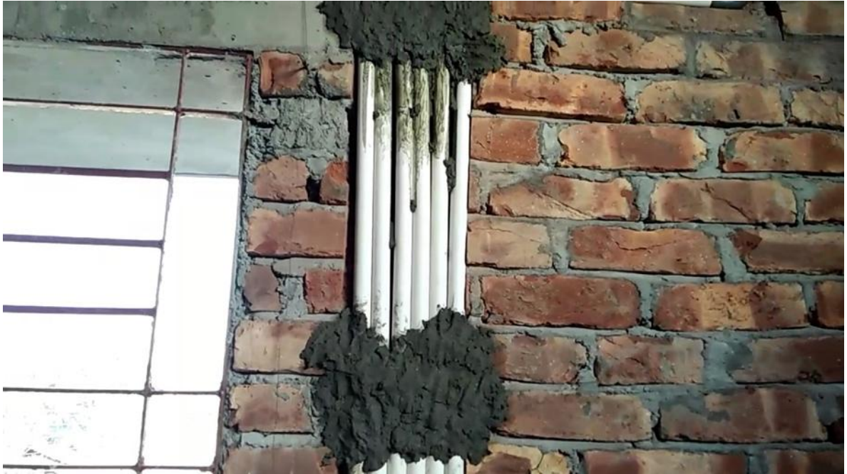
Concealed conduit and wires installation
