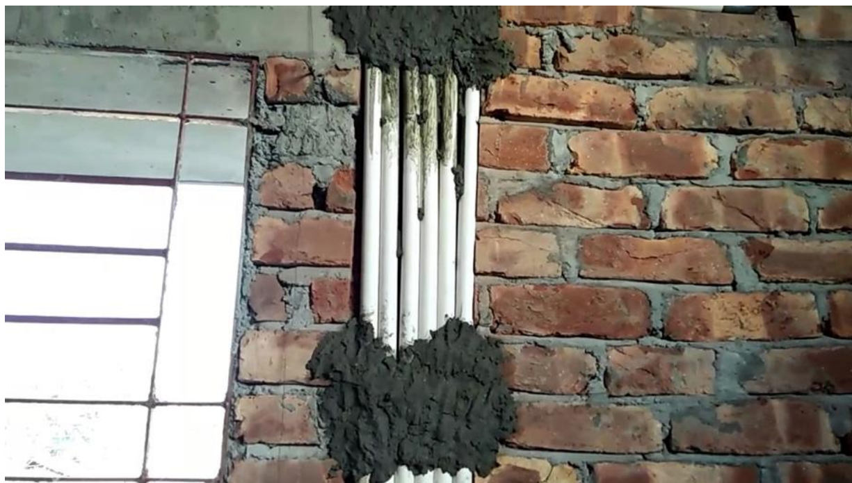
Concealed conduit and wires installation
