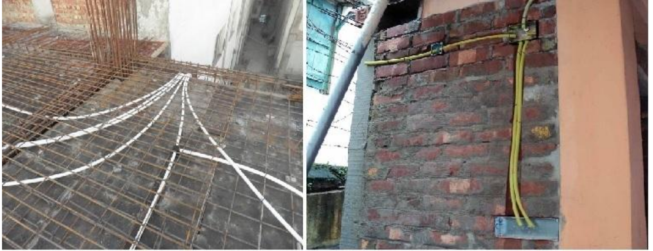
Concealed Conduit Installation in Slabs and Walls
